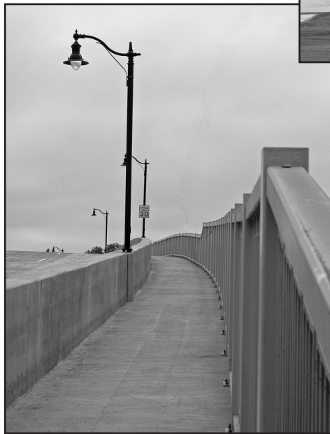
New lights, railings and walkways make the bridge pedestrian and bike friendly.
