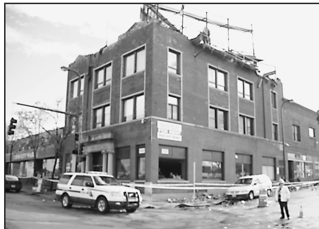
42nd Avenue Station, window blown out, billboard on roof blown off tearing off bricks from the building.
